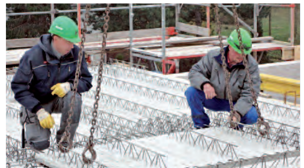
▶ Betondeckenelementmontage in Berlin-Spandau
