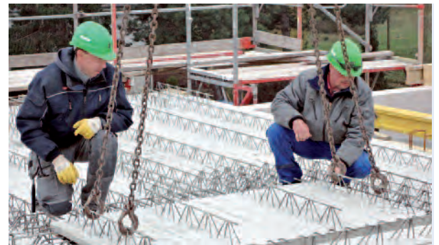
▶ Concrete ceiling element assembly in Berlin-Spandau
